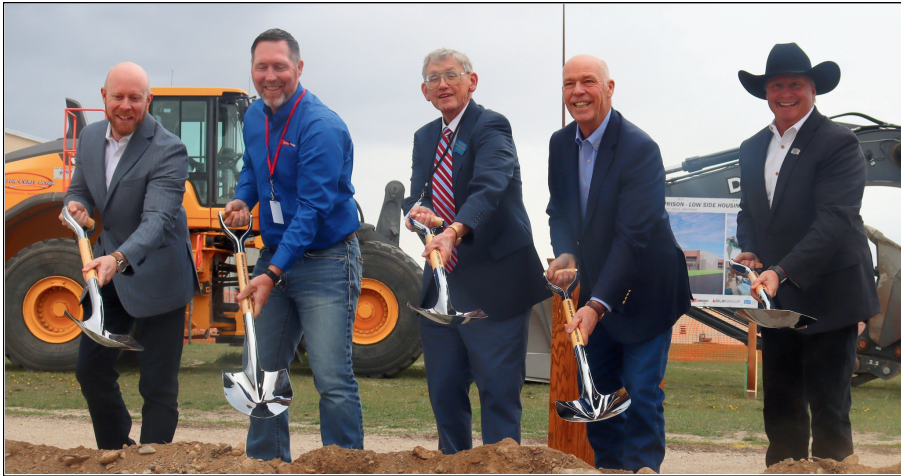
Governor Greg Gianforte and DOC Director Brian Gootkin break ground in a ceremony to kick off the construction at Montana State Prison on the new low-side housing units.
